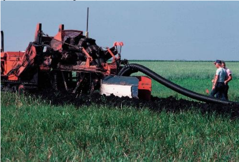
Figure 19. Installation of plastic tile to remove excess soil water.
